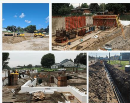
Construction progress, new peopleCare Tavistock LTC Home
